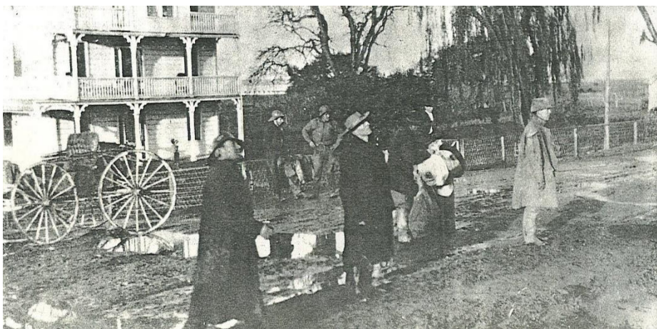
The Hart Fellows Smith home in Isleton during the 1907 flood
