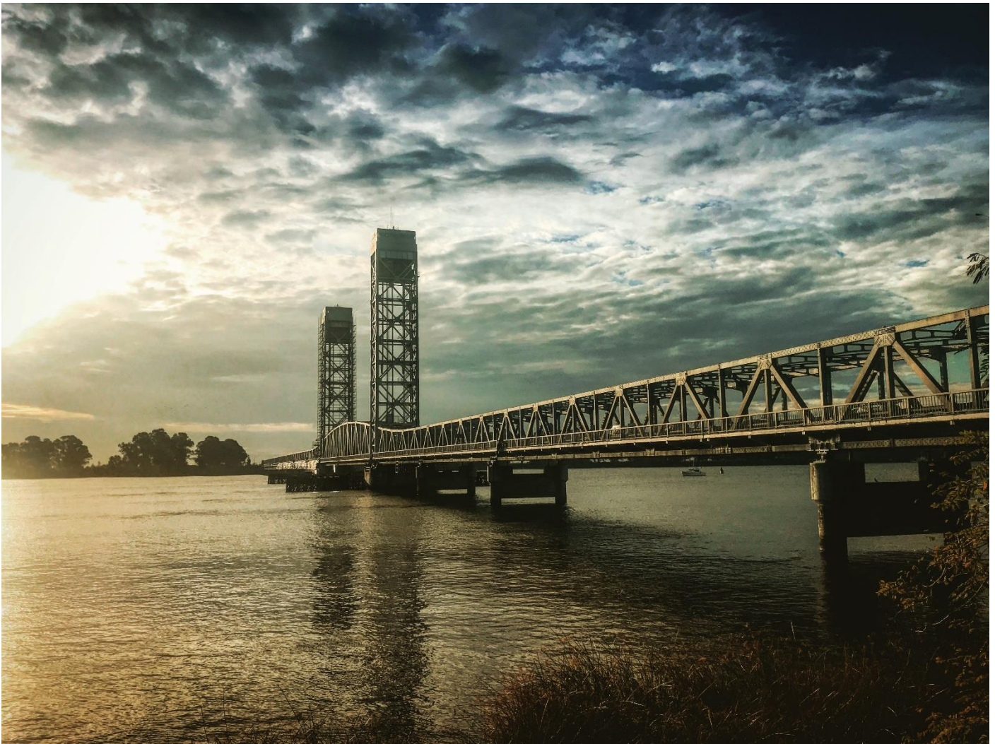
Rio Vista Bridge today. Photo courtesy of Gregory Mitchell/Rvbridgeman
