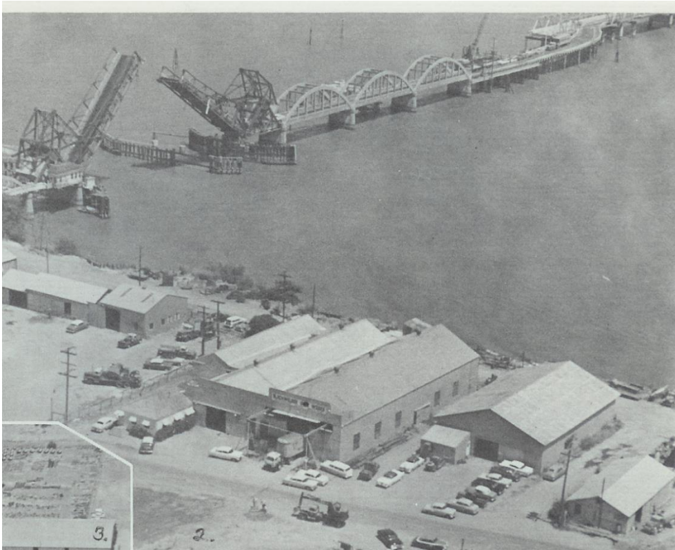
Old and new bridge construction, 1958
